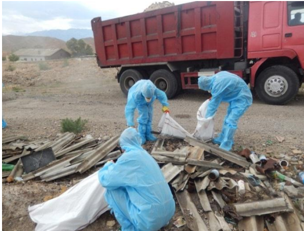
Training Practical asbestos disposal activities
